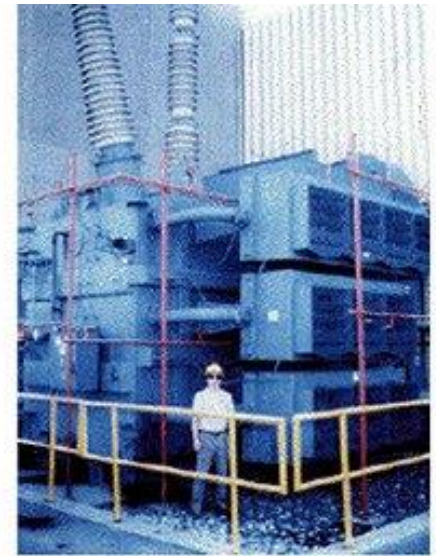
PJM Public Service Step Up Transformer Severe internal damage caused by the space storm of 13 March, 1989
